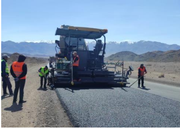
Photo 13. Asphalt paving. km 20+200. April
