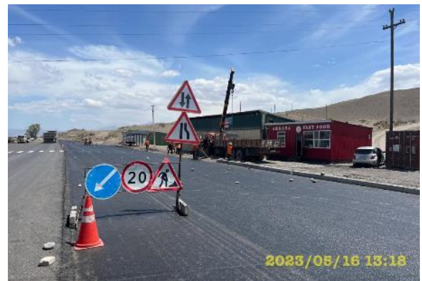
Photo 32. Installation of parapets km.81+200. May
