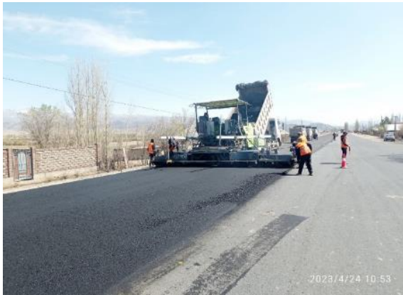
Photo 29. Paving the base course of ac pavement km 69+800-70+370. April
