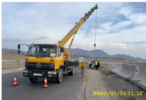
Photo 5. Lot 1. Installation of parapets km.22+850-22+970 LHS. January
