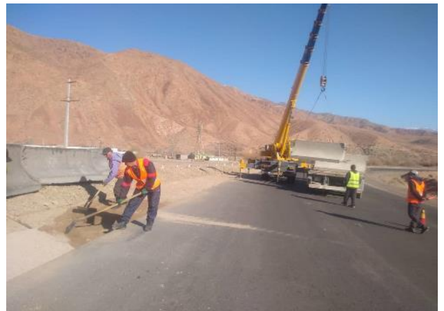
Photo 10. Lot 1. Installation of parapets km 14+300. March
