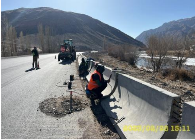
Photo 7. Lot 1. Assembly of installed parapets from km 14+000-15+000. February
