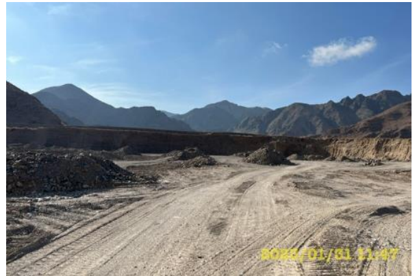
Photos 62 and 63. Lot 1. Quarry km 16+600. It is required to bring stability of quarry sides to a safe condition, i.e. the angle of inclination of quarry side should be equal to 70° (not more).
