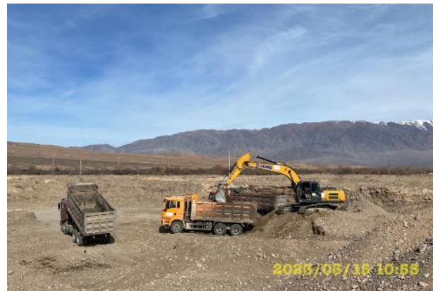
Photo 58. March. Quarry development at km. 9+000.
