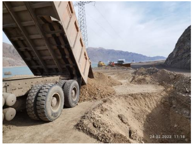
Photo 8. Lot 1. Earth works at km. 40+800. February
