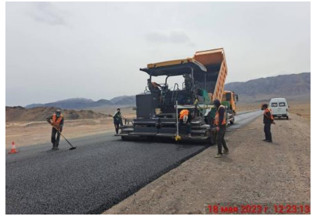
Photo 16. Laying asphalt. May
