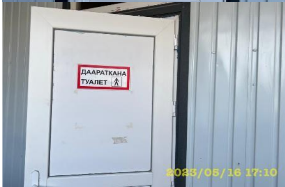
Photo 43. Lot 1. Women's and men's toilets.
