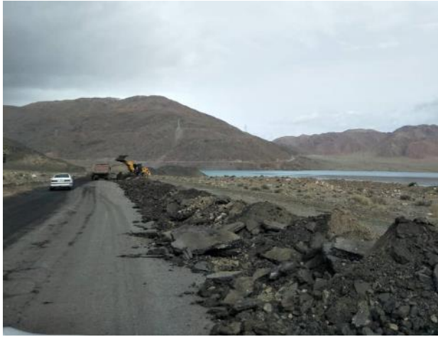
Photo 19. Scarifying of old asphalt. Km 39. May
