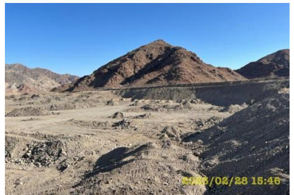
Photo 65. Quarry sides of km.16+600 have been brought to a safe condition
