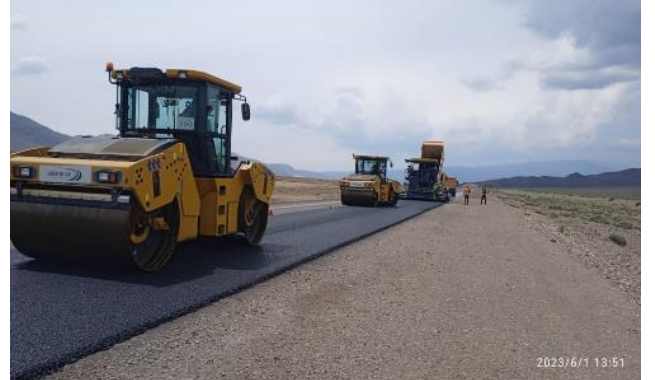
Photo 22: SMA paving, km.25+935--26+965 RHS. June
