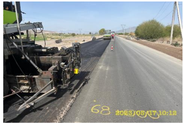
Photo 30. Paving the base course of ac pavement km 68+000. May
