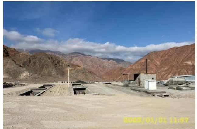
Photo 56. Reinforced concrete production site. Sanitary condition of territory is satisfactory. January.
