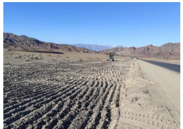
Photo 67. Bypass road at km. 22+000-23+000. Reclamation has been carried out.
