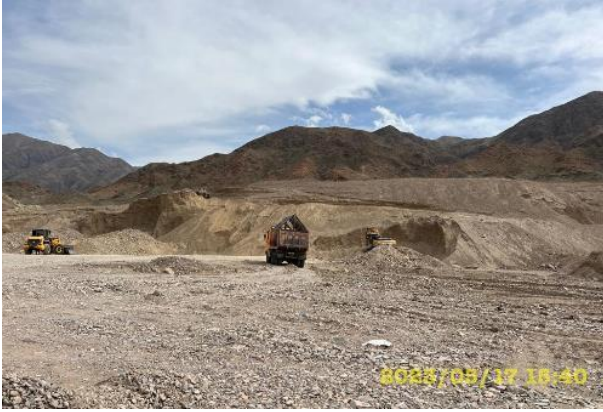
Photo 61. Quarry development at km. 34+240. May
