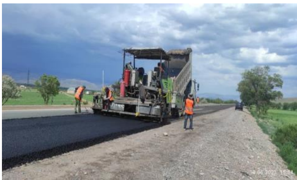
Photo 33. SMA Arrangement km 78+120-km 79+100 LHS. June
