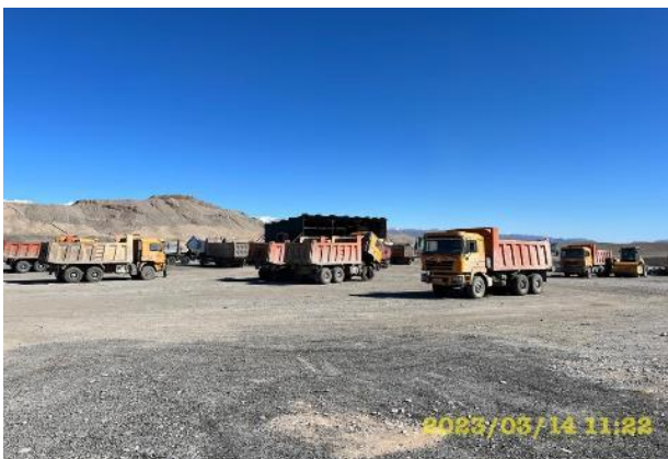
Photo 80. March. Sanitary condition of the construction equipment parking area is satisfactory, no oil pollution was observed.
