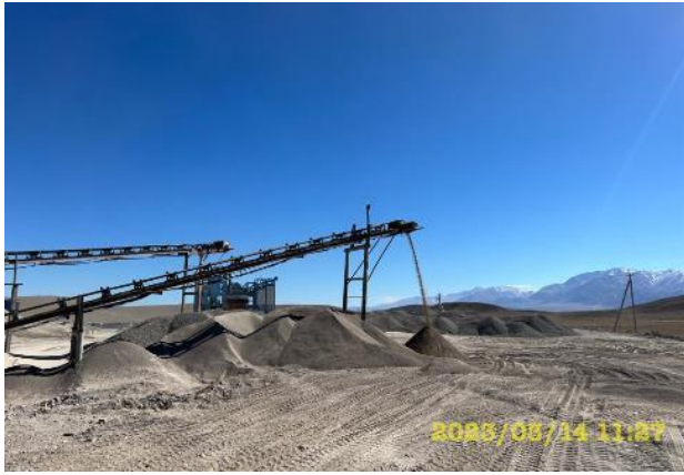
Photo 88. Preparation of construction materials at Crusher. March
