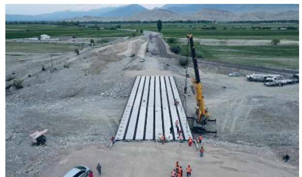
Photo 34. Bridge km. 65+410, installation of slabs. June
