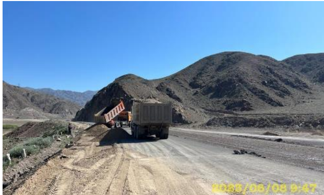
Photo 21. Earthworks: km.42+000-43+000 June
