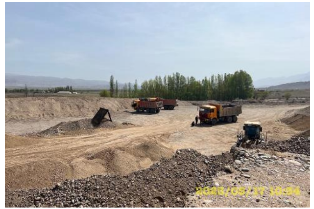
Photo 89. Quarry development km.75+400. May
