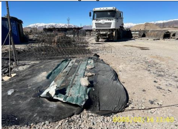
Photo 92. Lot 2. Reinforced Concrete Production site. Bitumen spill.
