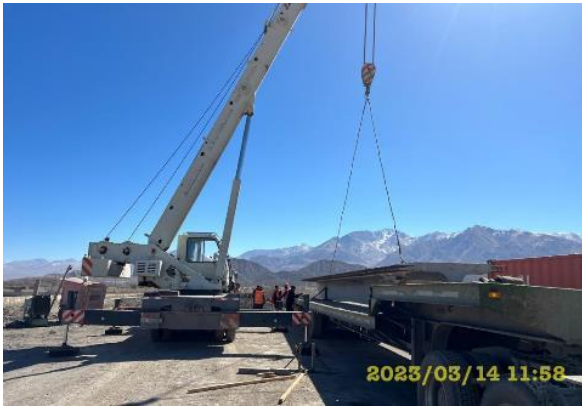
Photo 27. Bridge installation km. 65+360. March
