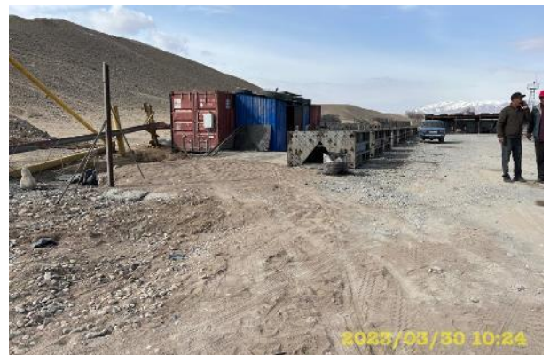
Photo 93. Lot 2. Reinforced Concrete Production site. After cleaning from bitumen spills.
