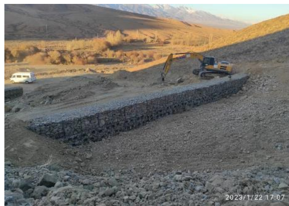
Photo 6. Lot 1. Erection of gabion km.12+795 LHS. January
