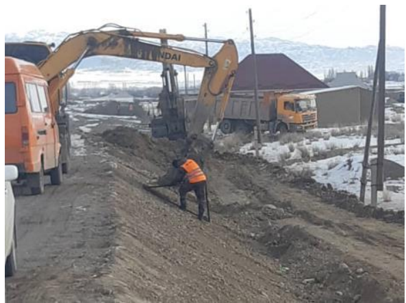
Photo 26. Slope cutting km 88+500-88+600 LHS. February
