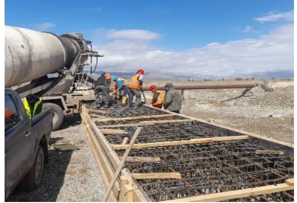
Photo 28. Pouring of monolithic cross beam of the abbatment no 4. April
