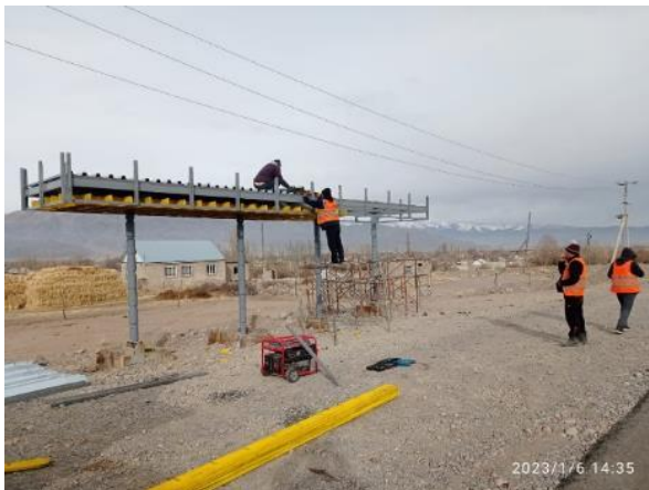
Photo 25. Constructing bus stop shed km 86+782 RHS. January
