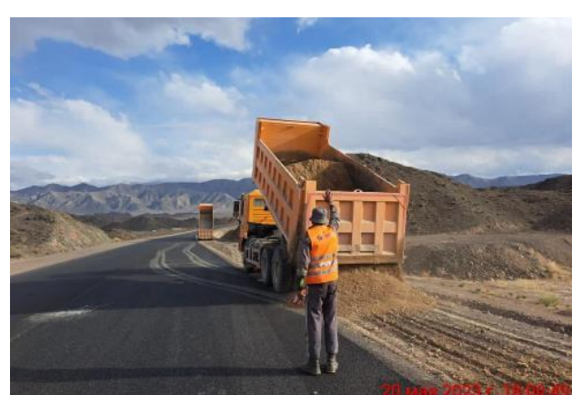
Photo 18. Construction of road shoulder km. 20+500. May
