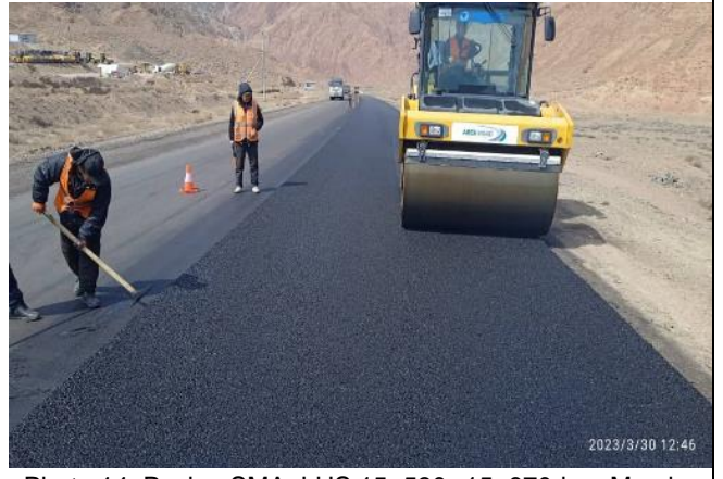
Photo 14. Paving SMA. LHS 15+530--15+870-km. March
