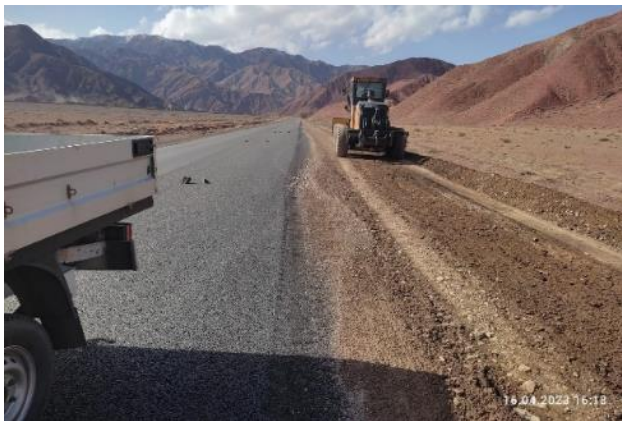
Photo 11. Earthworks: road shoulder leveling. Km. 18+500. April
