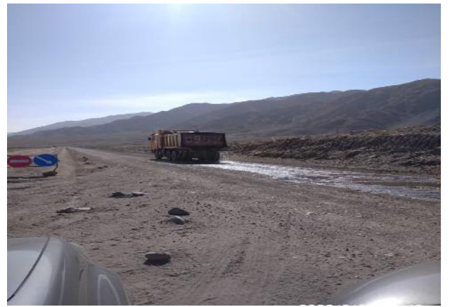
Photo 69. Lot 1. Hydro-irrigation of unpaved road sections at km. 37+000-38+800
