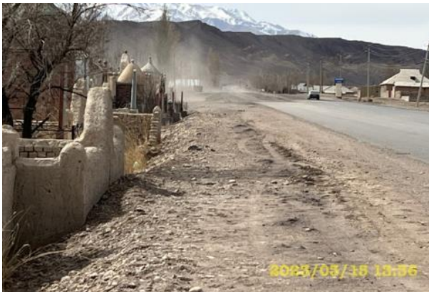
Photo 86. Lot 2. March The cemetery km 68 road LHS not fenced and close proximity to road: as a result of roadside construction, some sections of grave fence have been filled with soil
