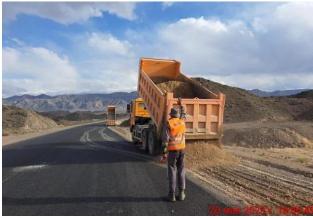
Photo 15. Constructing road shoulder km. 20+500. May
