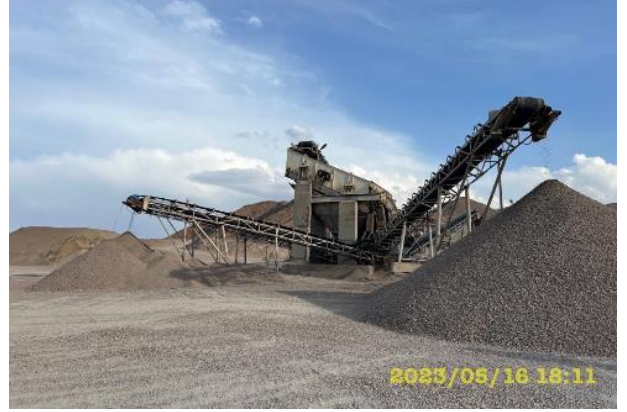
Photo 62. May. Material preparation at Crusher plant.
