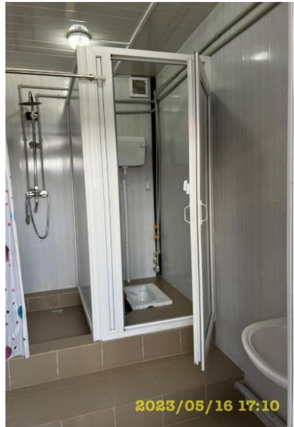
Photo 44. Lot 1. Women's toilet and shower room
