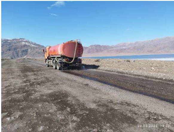
Photo 9. Lot 1. Hydro-irrigation of unpaved road sections km. 41+000-43+000. February
