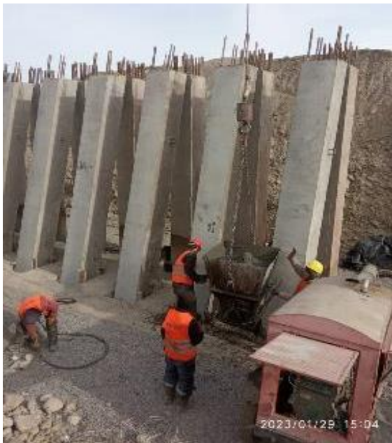
Photo 23. Bridge km 65+410. Reinforcing of piers with foundation. January
