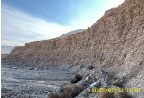
Photos 62 and 63. Lot 1. Quarry km 16+600. It is required to bring stability of quarry sides to a safe condition, i.e. the angle of inclination of quarry side should be equal to 70° (not more).
