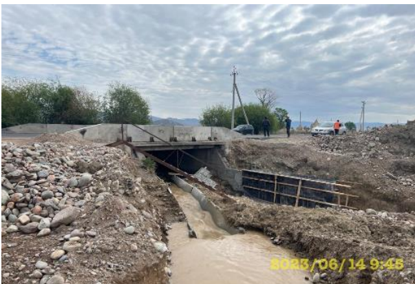
Photo 108. Mukandyn-Suusu river bridge, km. 68+040 It is necessary to provide protective measures to prevent soil from entering the river during construction works.
