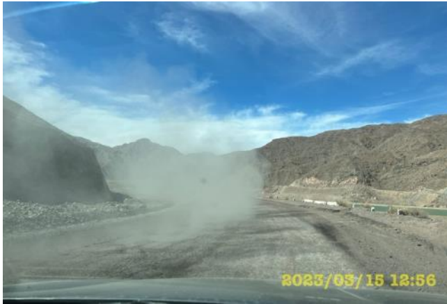
Photo 68. March. Dust on the unpaved road section at km. 37+000-38+000
