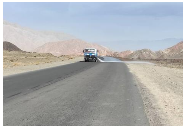
Photo 12. Watering of pavement km. 19+700. 07.04.2023.
