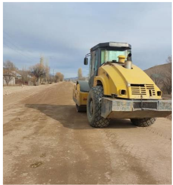
Photo 24. Compaction of subbase layer (2nd layer) km 70+340-70+740 RHS. January
