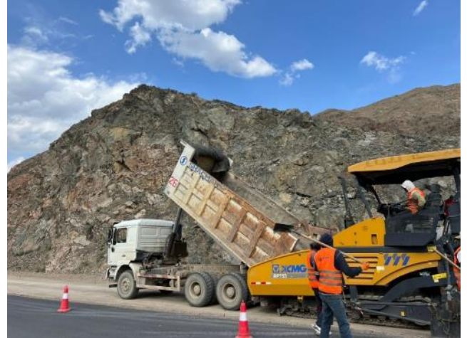
Photo 20. Base paving. 42+000-42+920 LHS. June
