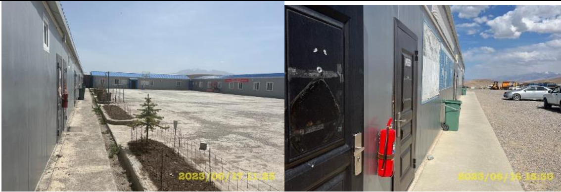
Photo 51. Offices and rooms for accommodation in the Contractor's camp
