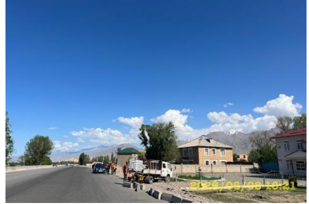
Photo 36. Installation of curbs. v. Kok-Jar. June.
