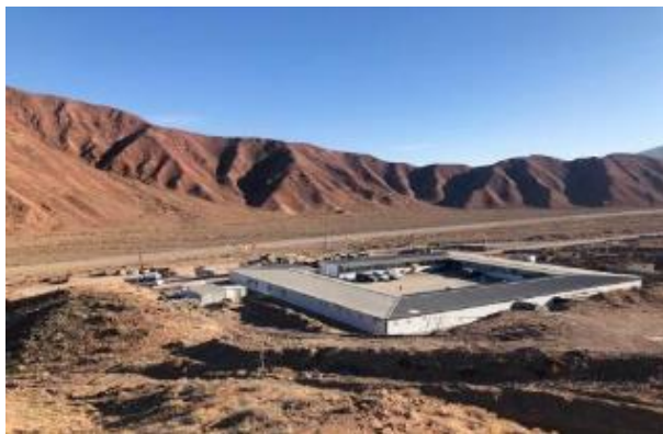
Photo 37. General view of camp Lot 1 km 16 + 100 (RS).
