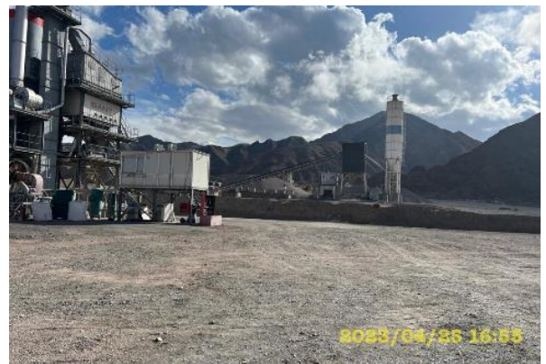
Photo 60. April. Sanitary condition of the industrial base territory is satisfactory. no oil product pollution was observed.
