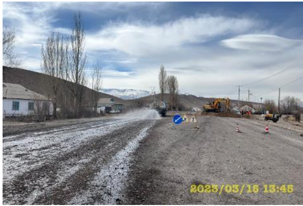
Photo 100. Hydro-irrigation of unpaved road sections at km. 69+840-71+000.
