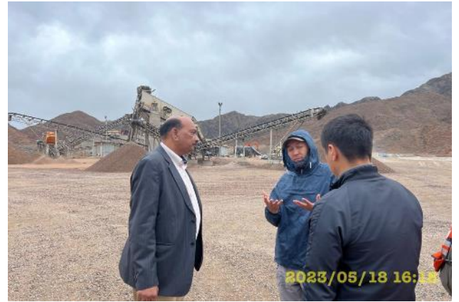
Photo 71. ADB Mission. Lot 1. Production base. Crusher plant
