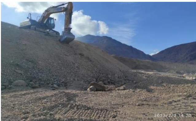
Photo 64. Quarry km 16+600. Work is underway to ensure stability of quarry sides.
