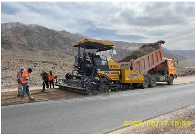
Photo 17: Earth works: km.38+000-42+000. May
