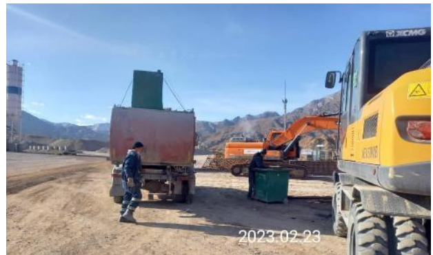
Photo 119. Lot 1. Solid waste removal from production base
