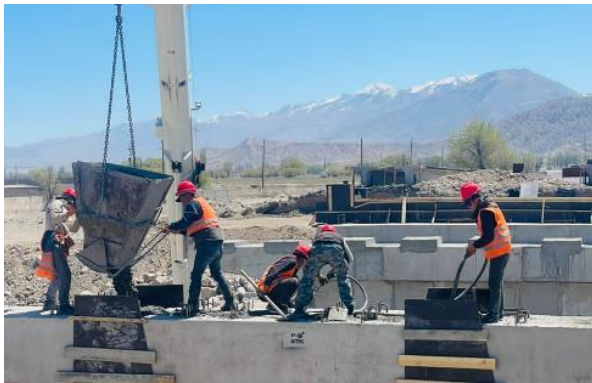
Photo 31: Bridge km. 65+410. Monolithic concrete, cross beam connection. May
